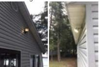
9. Marginal Exterior Electric Outlets: 110 VAC - all exterior outlets should be covered and GFCI protected for safety as they are exposed to water
