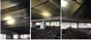
7. Marginal Piers/Posts: Block - block supports have movement noted and repair is needed, monitor and repair supports before damage is done to the building which will be difficult to recover from, supports and movement were discussed
